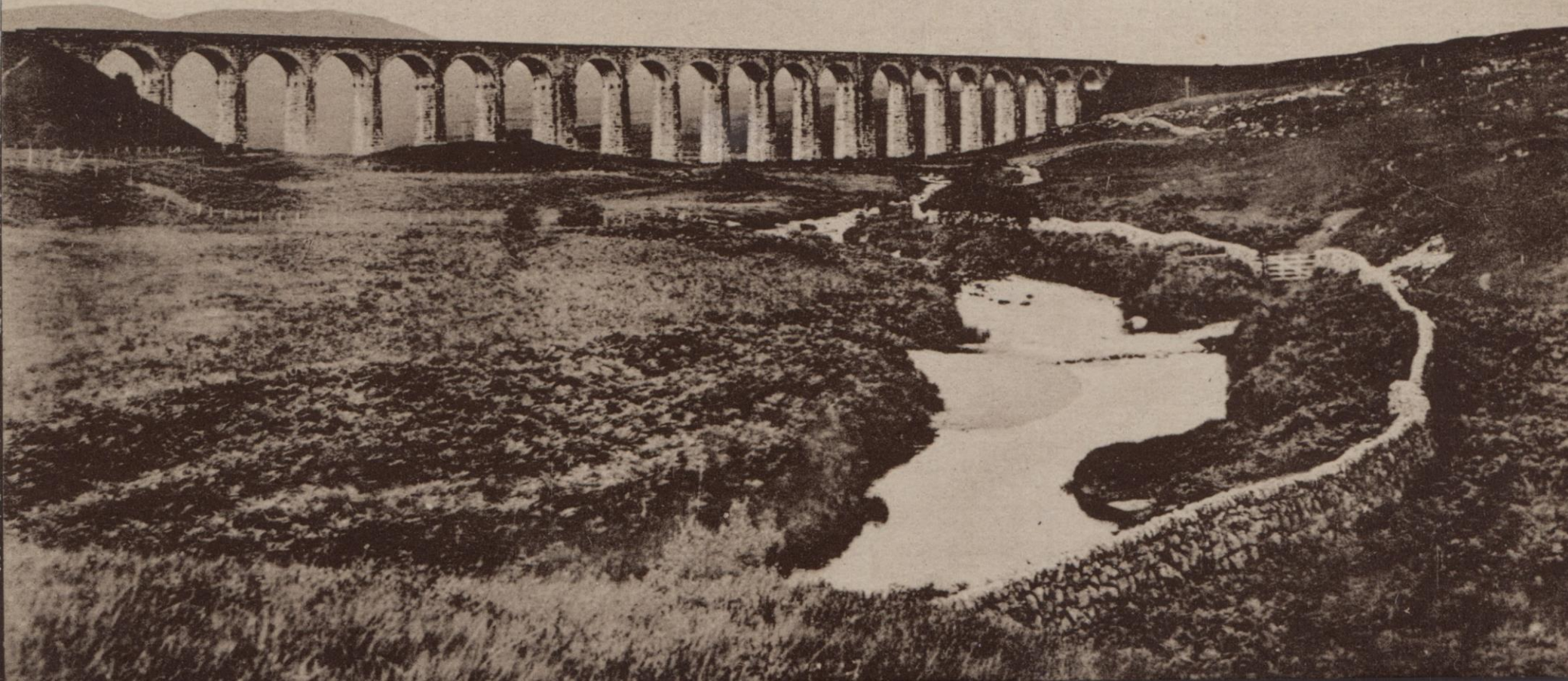
16.24 Big Water of Fleet Viaduct before re-inforcement
